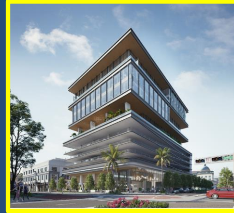
300 Banyan In Construction
