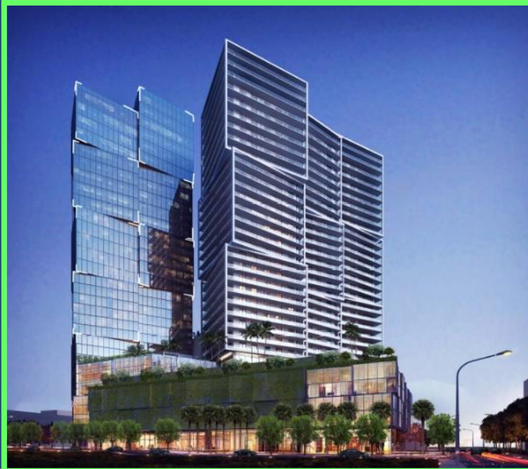
One West Palm Construction underway 200 rooms
