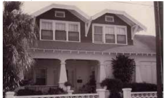
Home of Henry Speed (demolished, property now owned by CRA), pioneer and land donor for Pine Pine Ridge Hospital. (Courtesy FMSF)
