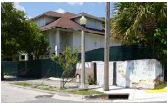
The property wall exists in part and can be used to match the texture and dimension of a new knee-wall or a full height wall.
