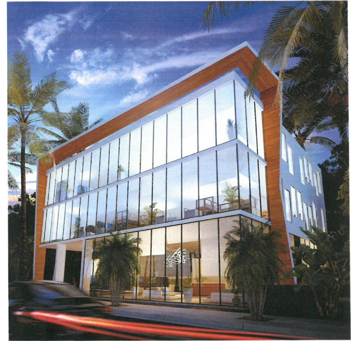
BUILDING 2 VIEW FROM S. DIXIE HIGHWAY 1/17/2015
