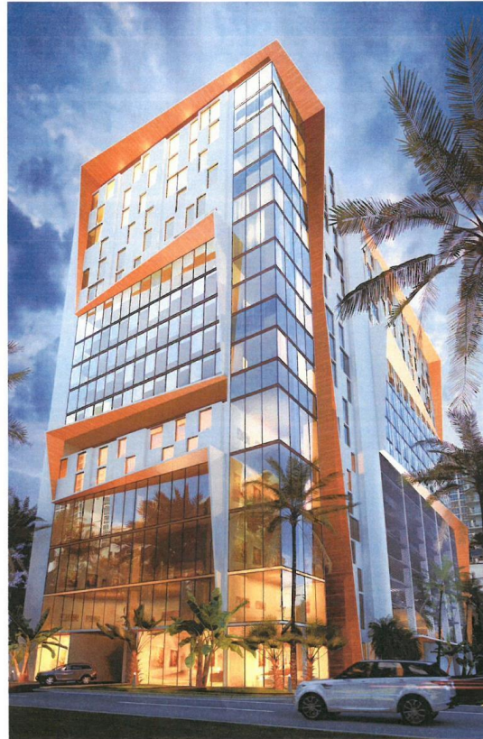
BUILDING 1 VIEW FROM S. QUADRILLE BLVD. 1/17/2015
