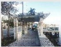
12 Flagler Trellis Replacement
