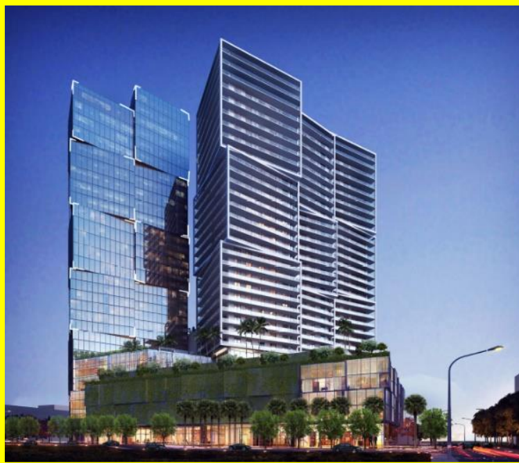
One West Palm Construction underway 200 rooms
