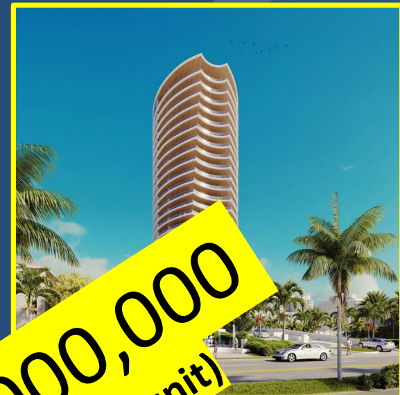
2 Forte Under Construction 1309 S. Flagler
