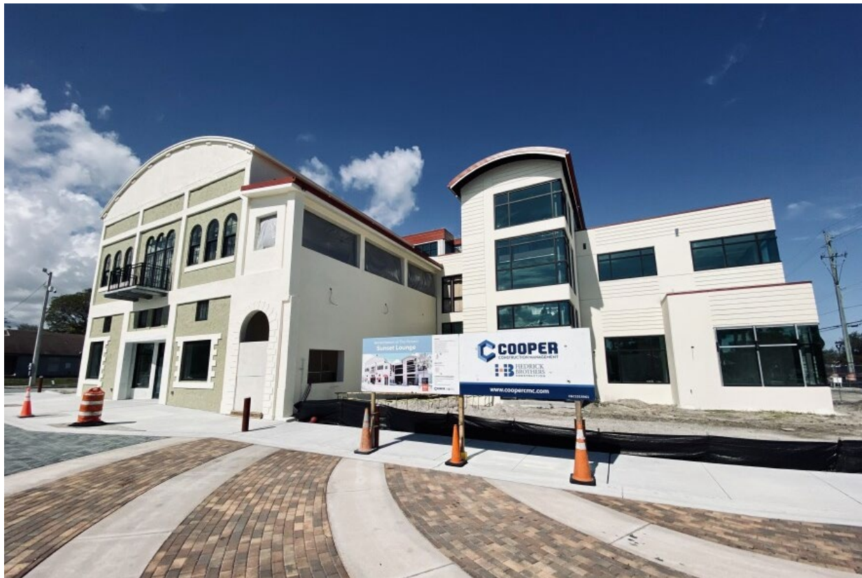
Sunset Lounge (under construction)
